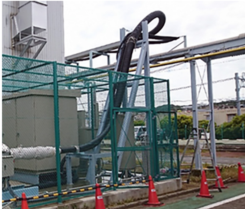
Bending parts of tri-axial superconducting cable, Courtesy NEDO
